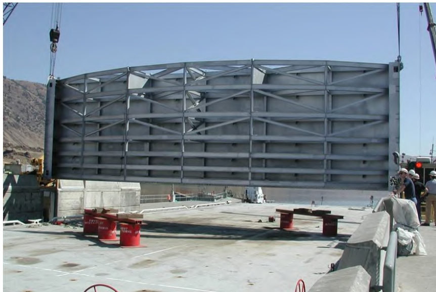
Figure 12-28. John Day Dam Vertical Lift Gate.
