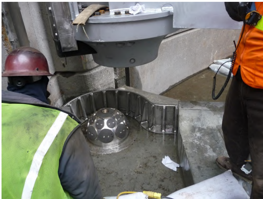
Figure 12-21. The Dalles Dam Miter Gate Pintle Installed.
