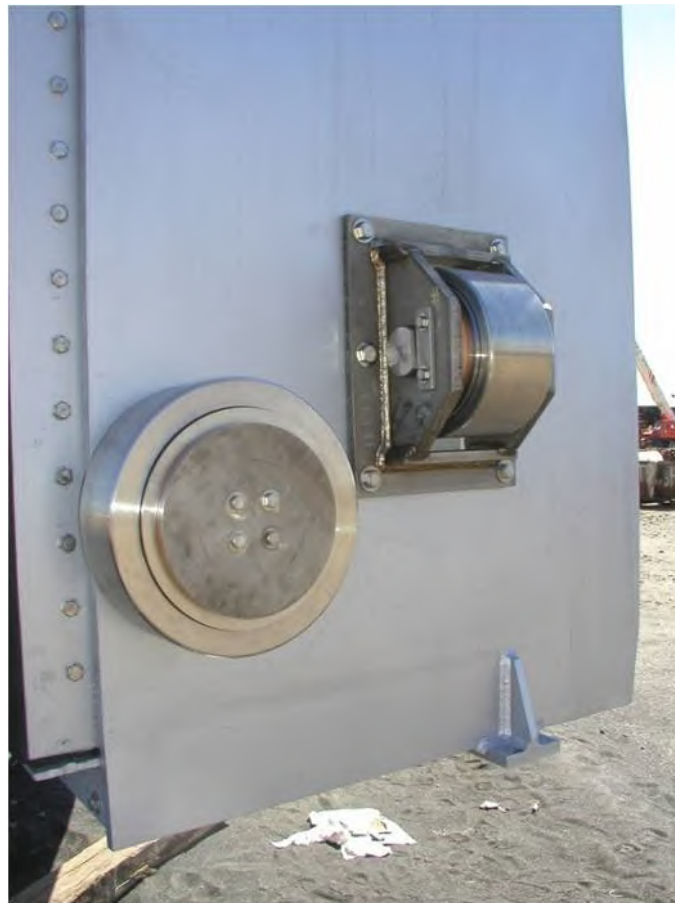
Figure 12-30. John Day Gate Bottom Guide Rollers (Self-Aligning).
