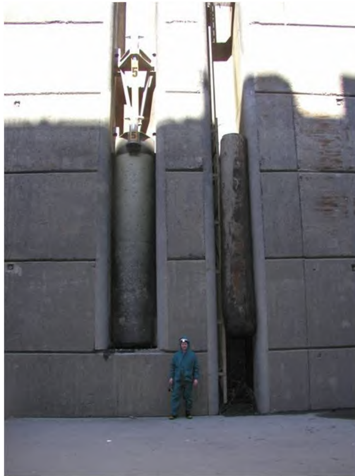
Figure 12-22. Bonneville Dam Floating Mooring Bit.
