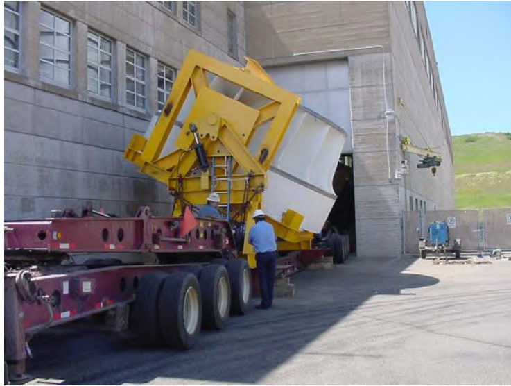
Figure 9-6. Francis Turbine Runner Transported into Powerhouse.
